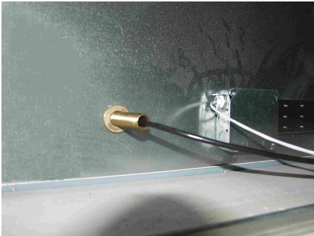
**Figure 19    Coaxial Cable Penetration of a Shielded Room**
