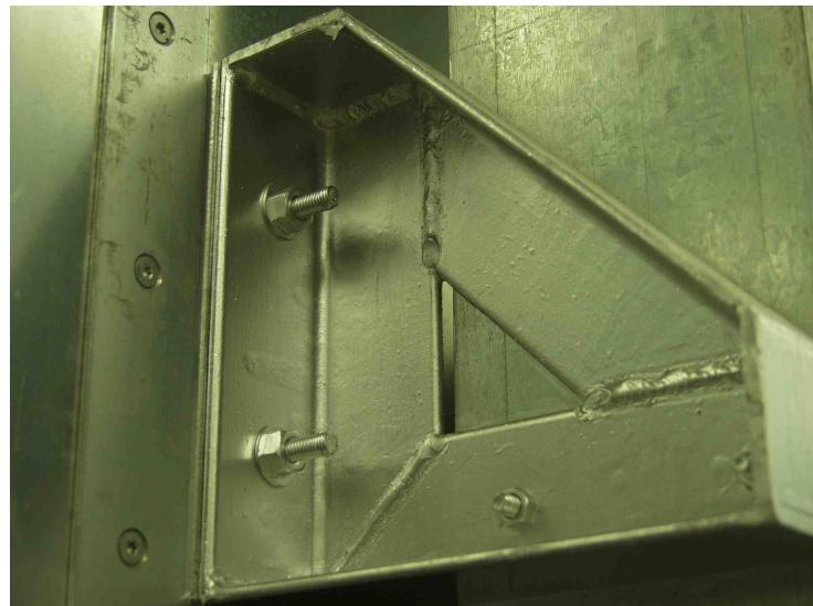
**Figure 54     Welds on Galvanized Metal Supports**
