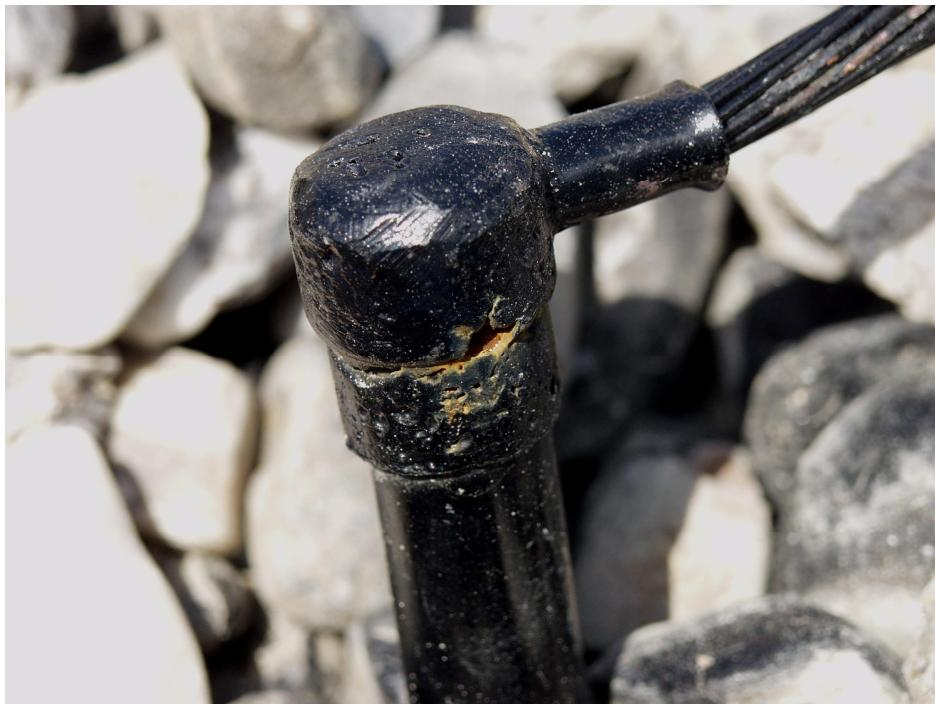
**Figure 15 CADWELD® on Antenna Counterpoise Wire**
