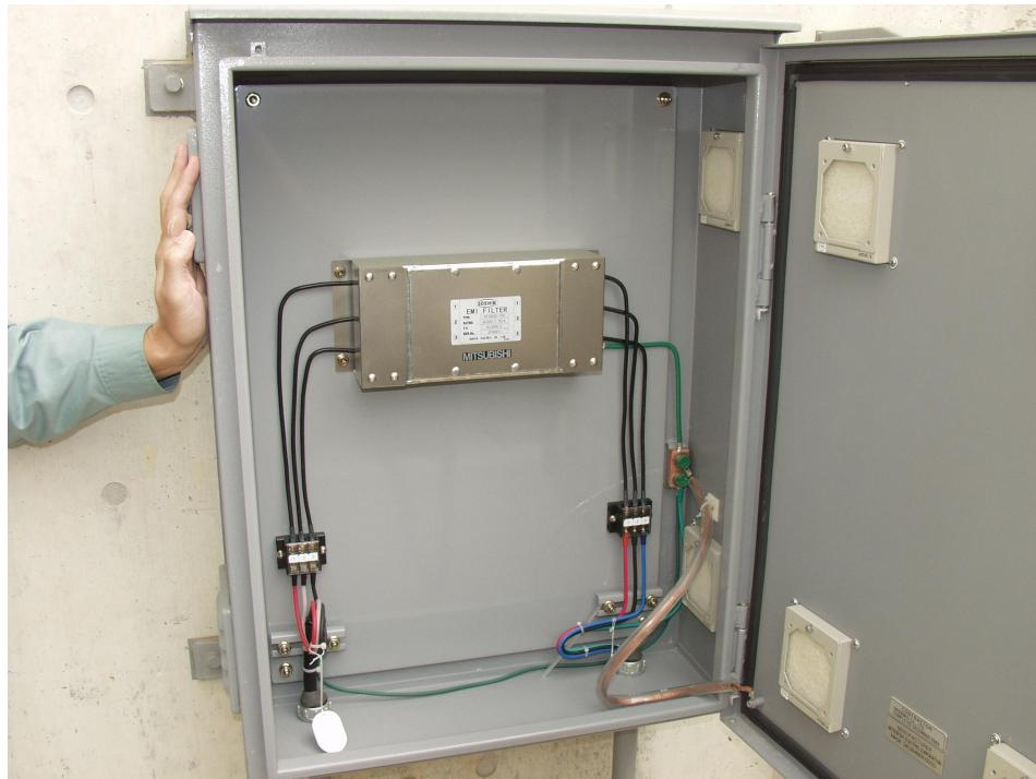
**Figure 49    Improper Filter Configuration**
