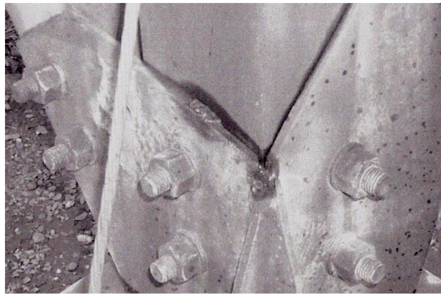
Figure 13    Weld on Galvanized Metal of a Receiving Antenna Tower
